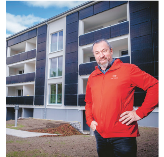
Energieautarke Mehrfamilienhäuser Self-sufficient apartment buildings
